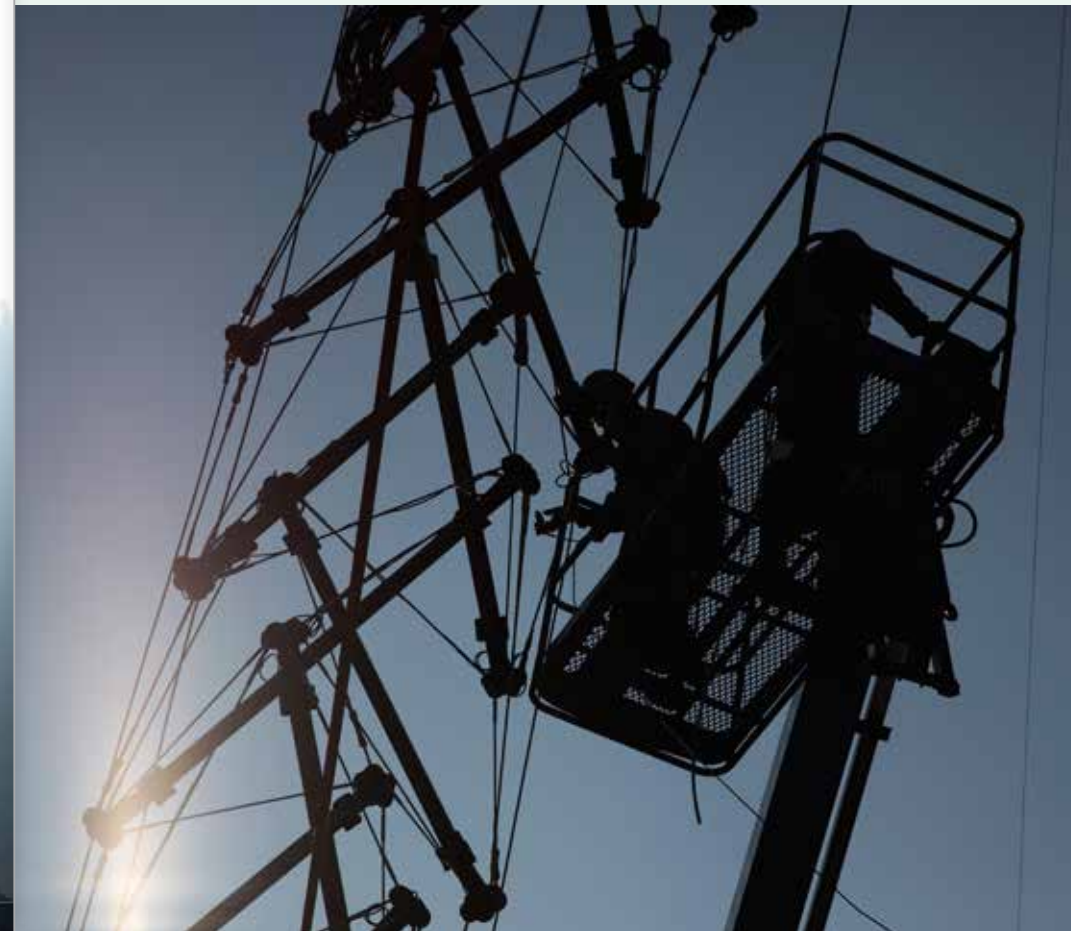
↑ Inox-Litze Toron Inox Stainless steel strand 1 x 19 E = 1,4 - 1,7 \cdot 10^5 \text{ N/mm}^2
